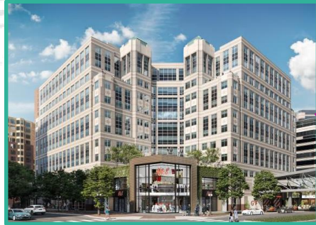
Ballston Exchange – Redevelopment of NSF building
