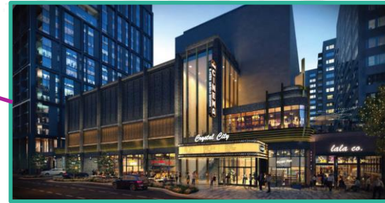
Central District Retail Ph I – 74,000 SF retail, Alamo Theater and grocery store
