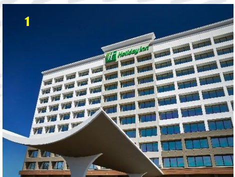
1 Renovated & repositioned hotel
