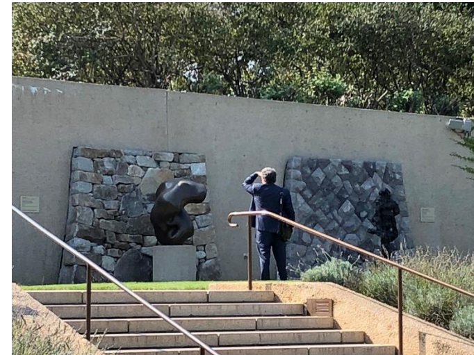
Mock-up Samples for Stone Walls
