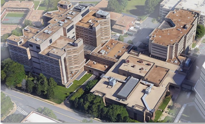
Adult Detention Center Security Upgrades
