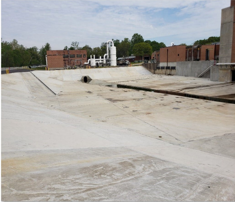
Noman M. Cole Pollution Control Plant Equalization Pond Rehabilitation
