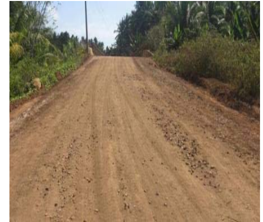
Road Construction Philippines
