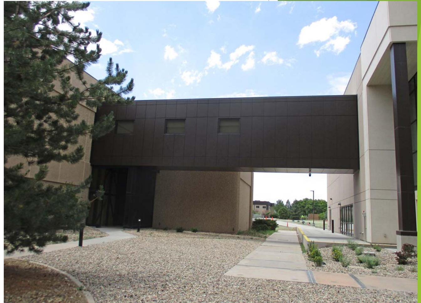
Secure elevated walkway connecting new Building 403 to existing Building 401 improves efficiency
