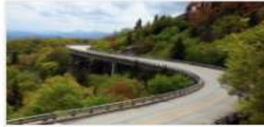
Park Facility Management Division (PFMD)
