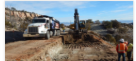
Major Construction Division (MCD)
