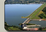
GAVINS POINT DAM/LEWIS & CLARK LAKE Total Storage: 0.43 MAF Total Flood Control Storage: 0.13 MAF 0.8% of System Flood Control Storage
