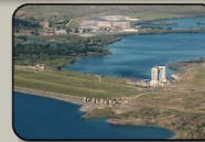
FORT PECK DAM & LAKE Total Storage: 18.46 MAF Total Flood Control Storage: 3.66 MAF 22.5% of System Flood Control Storage
