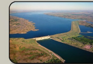
BIG BEND DAM/LAKE SHARPE Total Storage: 1.81 MAF Total Flood Control Storage: 0.18 MAF 1.1% of System Flood Control Storage
