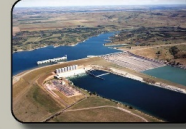
FORT RANDALL DAM/LAKE SHARPE Total Storage: 5.29 MAF Total Flood Control Storage: 2.29 MAF 14.1% of System Flood Control Storage
