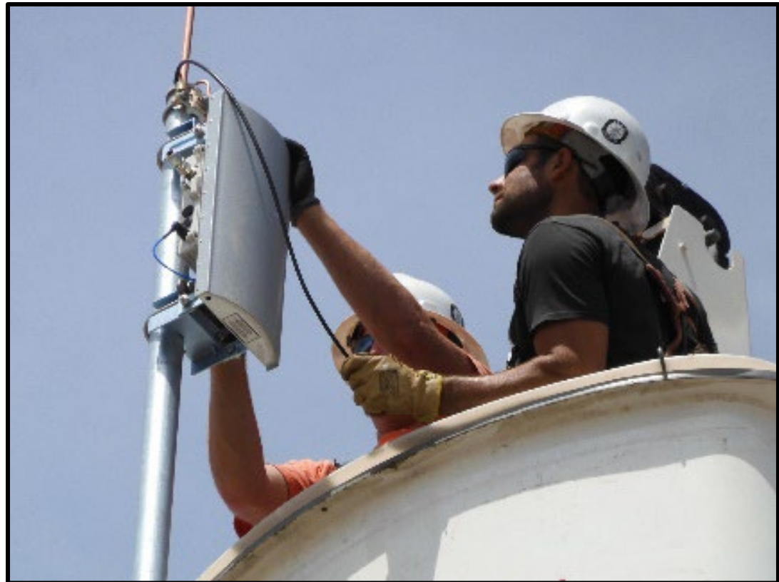
Munitions Storage Area Radio Replacement
