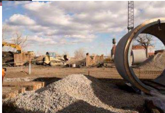
Targeted Sewer Separation
