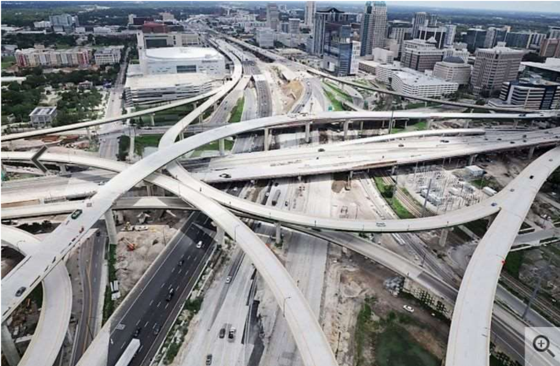
At the I-4 Ultimate project in Orlando, the Skanska-led joint venture construction team, SGL Constructors, has completed the critical State Road 408 (S.R. 408) portion of the 408/Interstate 4 (I-4) interchange, ahead of schedule.
