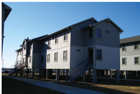
1995 Dining Facility expansion, Billeting (Bldg 501-507) and Classrooms (Bldg 509) built above flood levels
