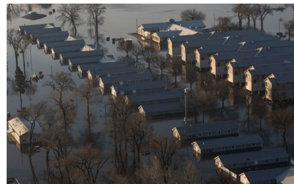
2019 Levee breach and significant flooding
