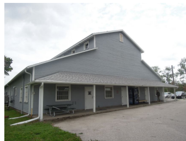
2014 Bldg 23 (Barn) renovated and conversion to HQ building
