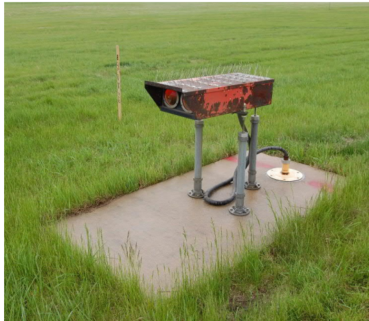
Deteriorated NAVAIDs
