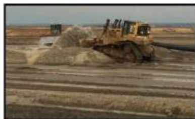
Center and left: The dredge line from the Dredge Iowa was pumping sand from the Missouri River into a containment and drainage system in the location of the land side seepage berm. Approximately 260K CY of sand was dredged into place in the levee footprint.
