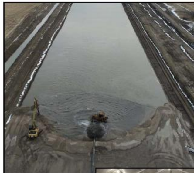
Center and left: The dredge line from the Dredge Iowa was pumping sand from the Missouri River into a containment and drainage system in the location of the land side seepage berm. Approximately 260K CY of sand was dredged into place in the levee footprint.
