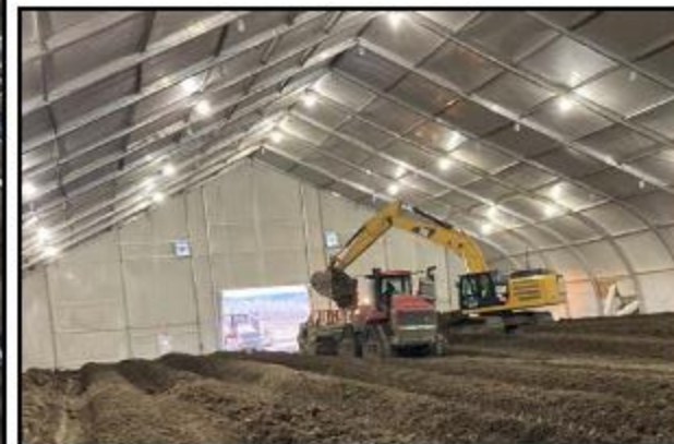
Above and bottom: Equipment conditioning and hauling cohesive material out of the heated tent structures setup during the cohesive material workable during freezing/winter conditions.
