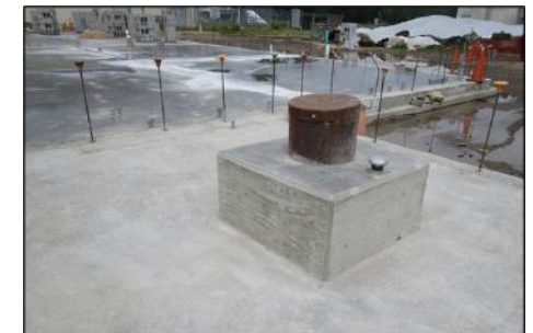
Completed Wellhead and Building Foundation
