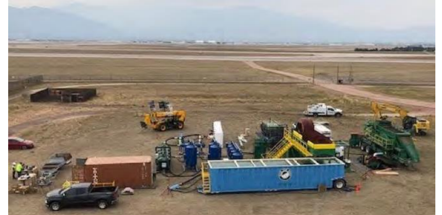
Soil washing system setup at site
