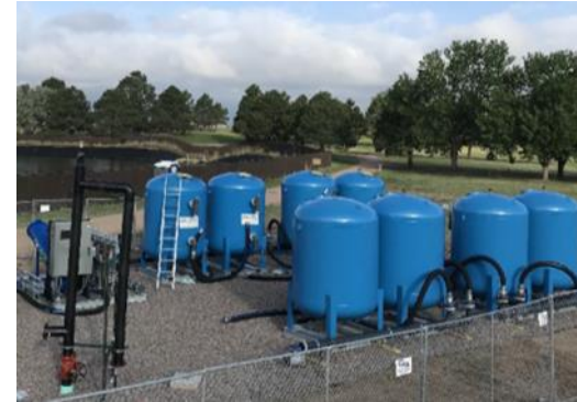
Above: GAC/IX treatment system for pond water
