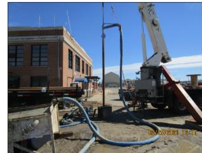
Drilling new 1,002 feet deep water supply well
