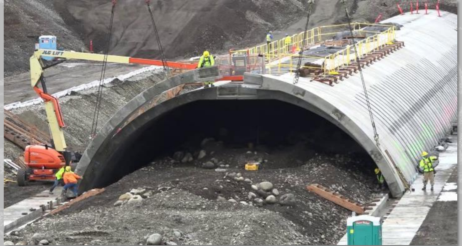
McChord Airfield Bridge Project
