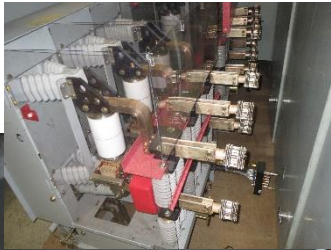
Circuit Breakers
