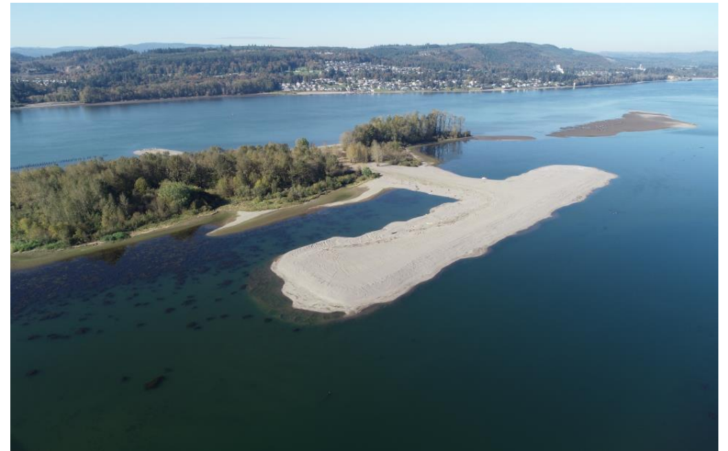
Woodland Islands beneficial use of dredged material (Photo courtesy of Columbia River Estuary Study Taskforce)
