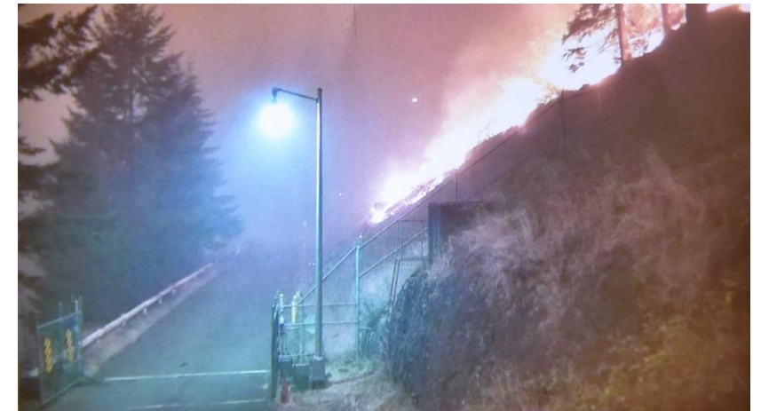
Fire Approaching Detroit Dam
