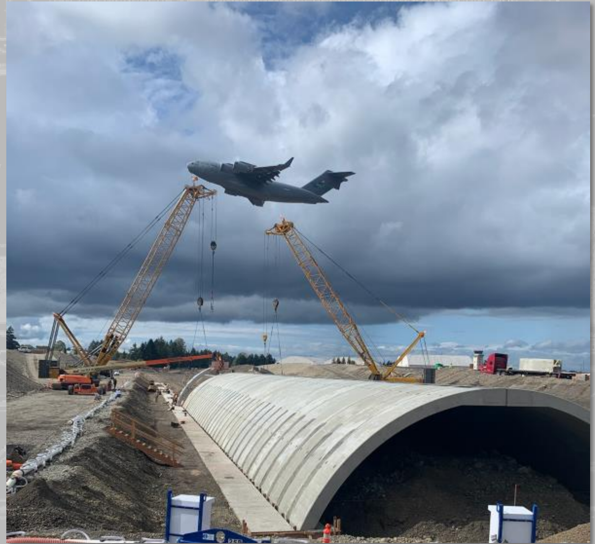
McChord Airfield Bridge Replacement
