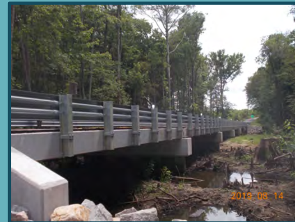
Completed bridge replacement project
