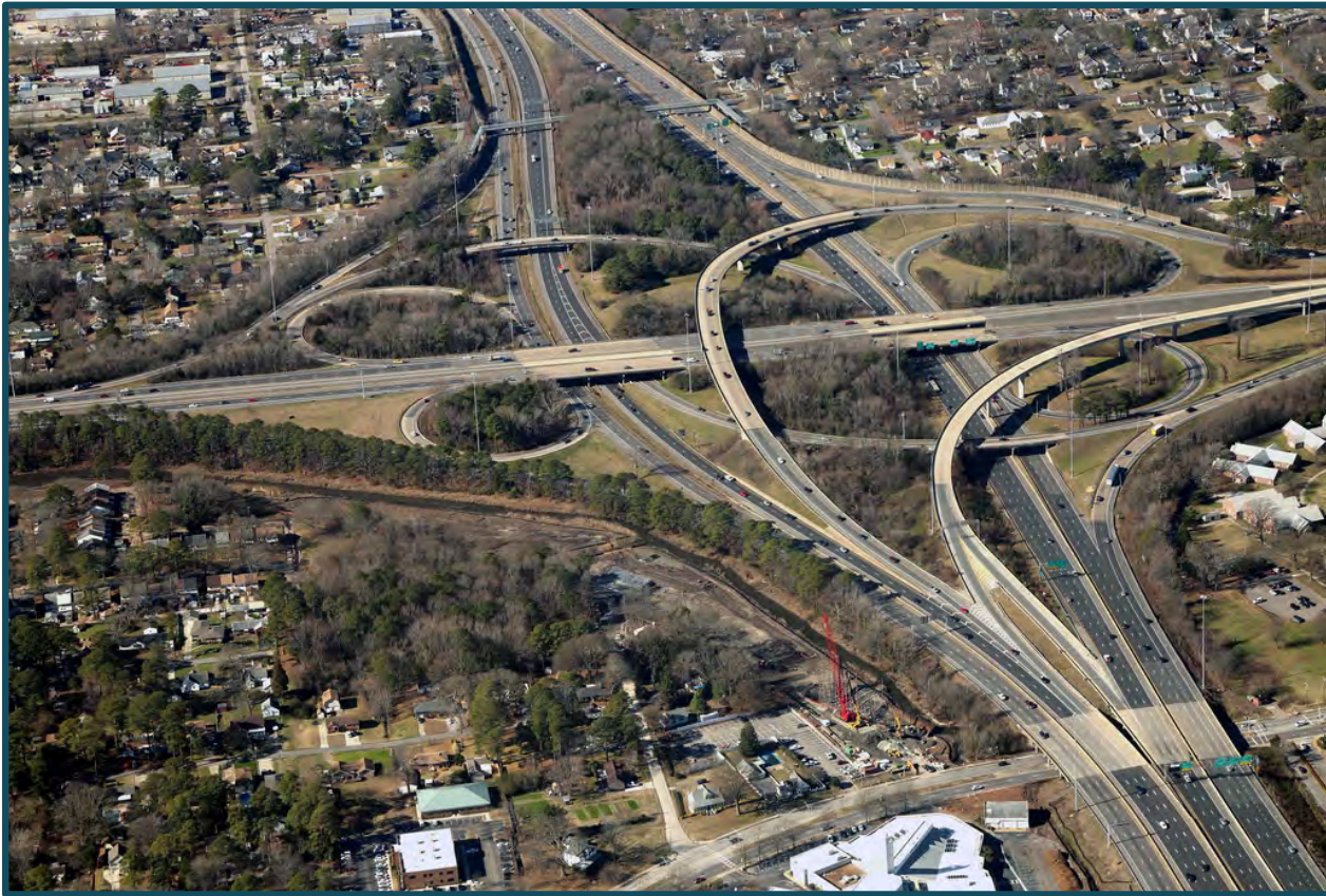
I-64/I-624 Interchange, Virginia
