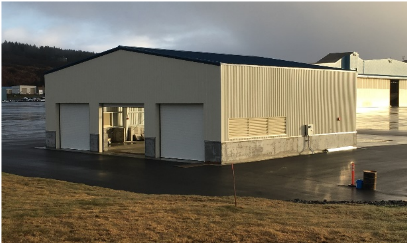
Liquid Oxygen Facility, Kodiak AK
