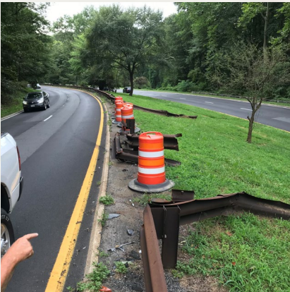
Current: Failed guardrail segments & patched roadway
