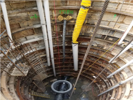
Sinkhole repair to 40-foot deep outfall
