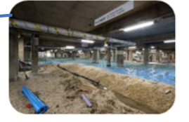
Garage Interior Rehabilitation, Phase 4, Rayburn House Office Building
