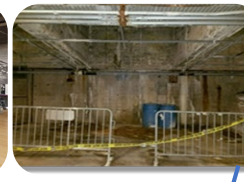
Garage Structural Repairs, JAB
