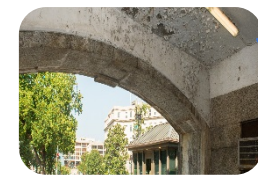
Senate Underground Garage Renovation Design-Build
