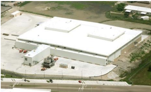
Dynamic Component Repair Facility, Corpus Christi Army Depot
