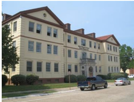
Building 5376 Renovation Barksdale AFB
