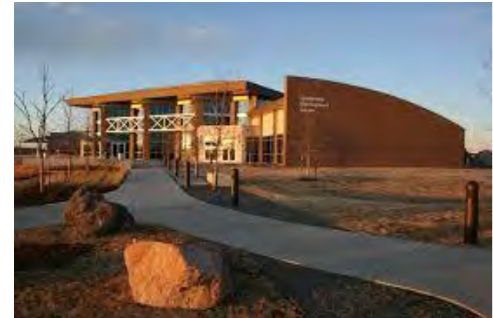
Leadership Development Center Buckley AFB, CO
