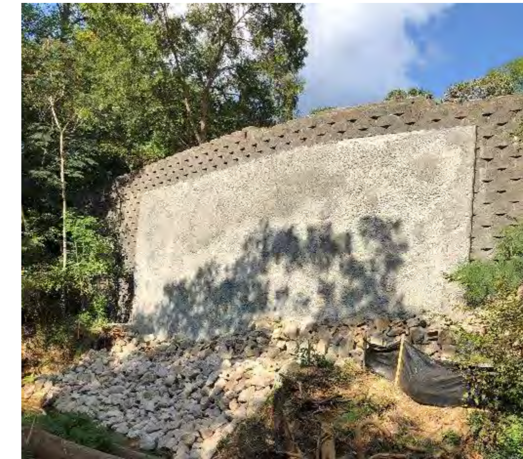
Retaining Wall Repair
