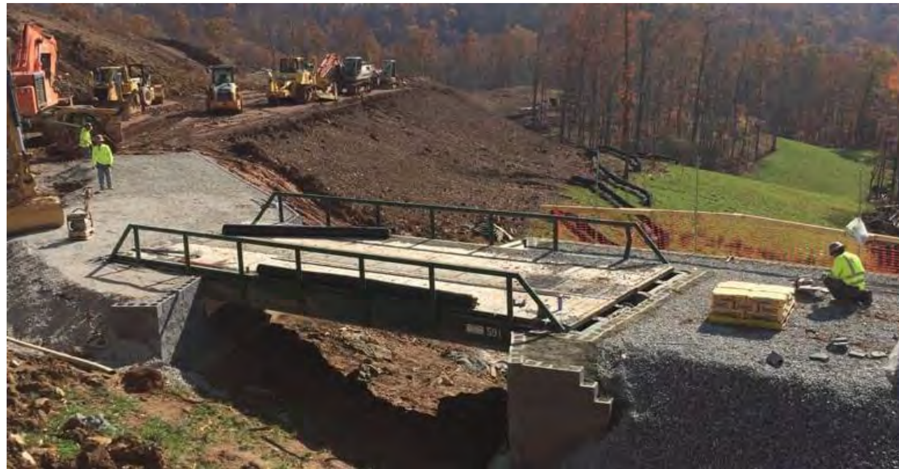
GCS Bridge Abutment Replacement
