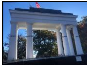
SAHNC Historic Gate Restoration
