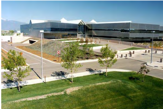
Air Force Space Command / Space Force Headquarters Renovation Peterson AFB, CO
