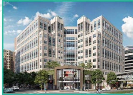
Ballston Exchange – Redevelopment of NSF building
