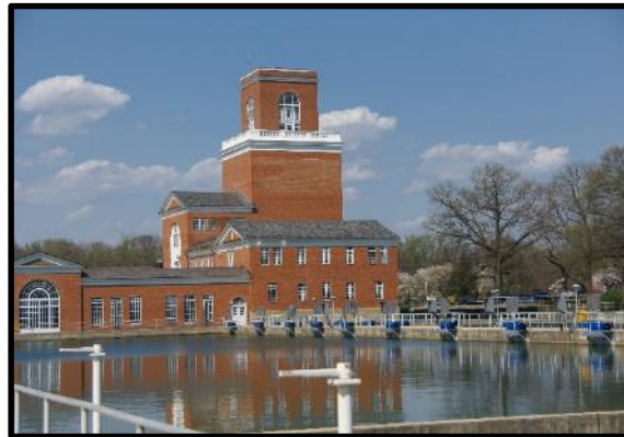
Dalecarlia Water Treatment Plant
