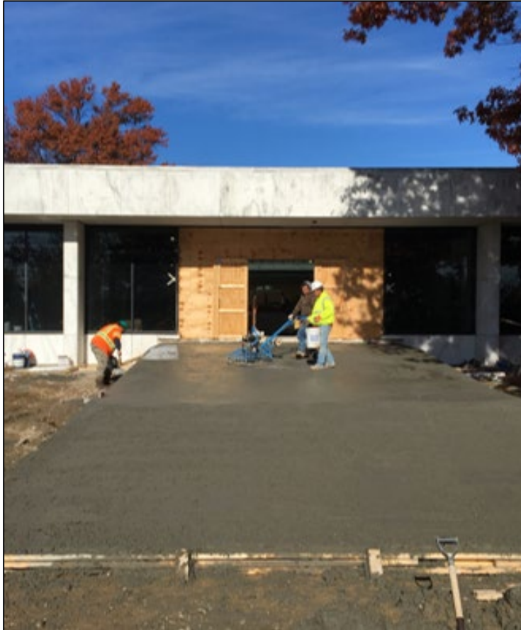
New Entrance Ramp (Dec 19)
