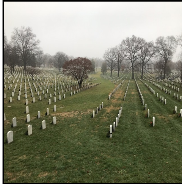
Section 47 Storm Drain Work Completed
