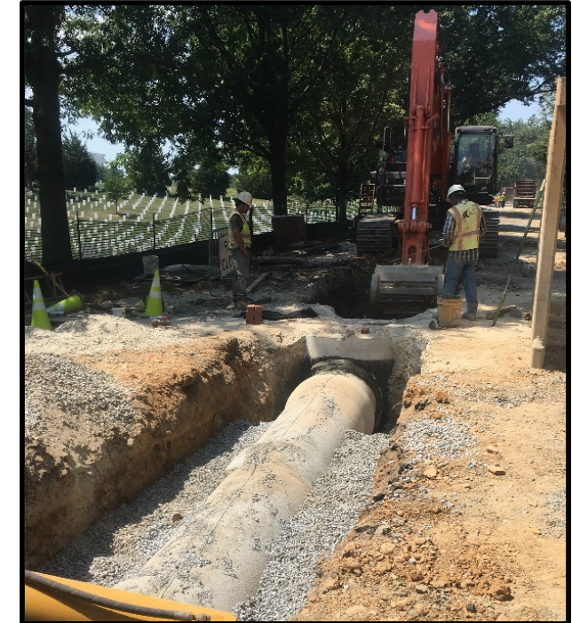
Grant Drive Structures and Pipe
