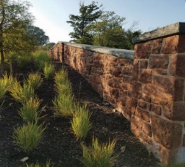
Boundary Wall Constructed of Reclaimed Materials
