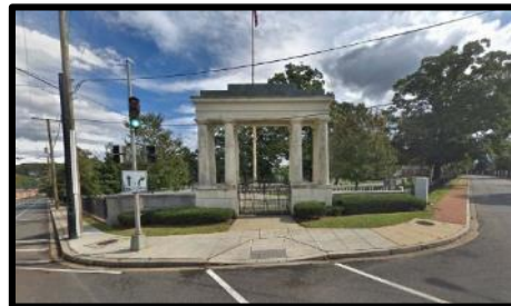
SAHNC Historic Gate Restoration
