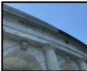
Memorial Amphitheater Renovation/Cleaning
