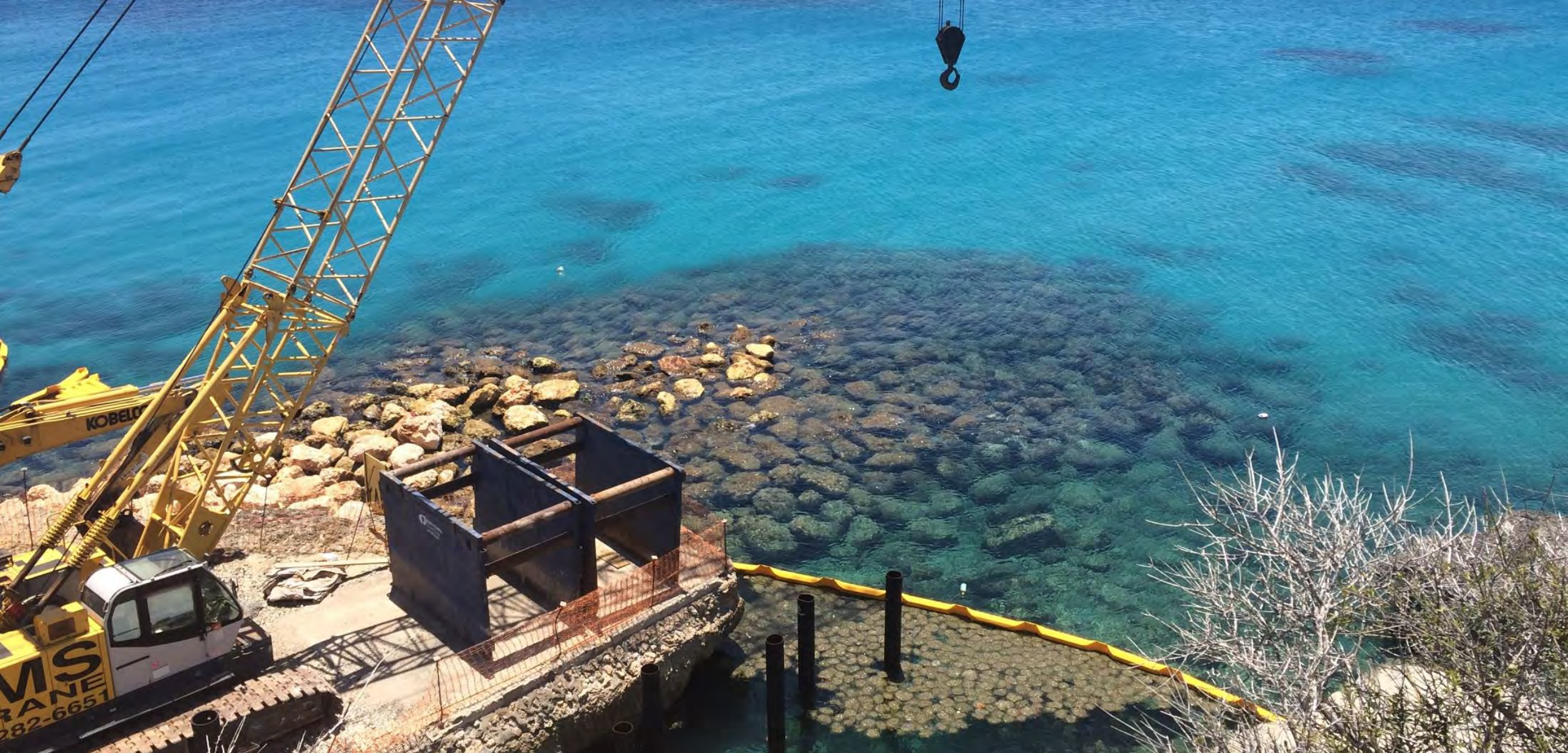
Guantanamo Bay Beach Repairs, NAVFAC
