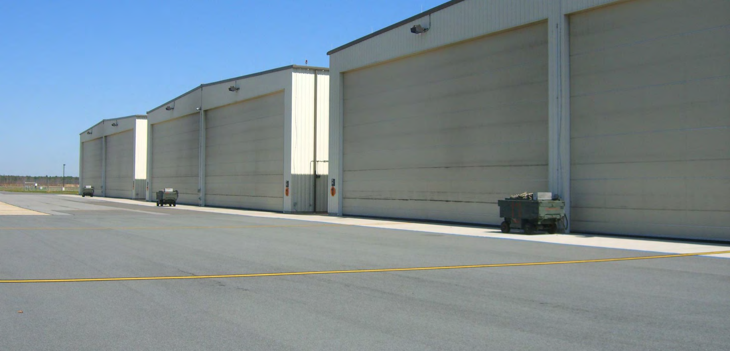
Aircraft Apron Repair, Atlantic City Air National Guard Base, NJ
