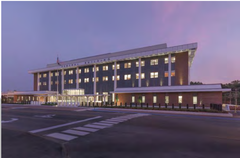
US General Services Administration, Margaret Chase Smith Federal Building + U.S. Courthouse Modernization + Expansion, Bangor, ME
