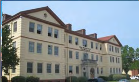
Barksdale B5376 Hangar B6426 NAVFAC Southeast
