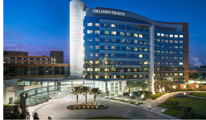
Orlando Health Orlando Regional Medical Center Expansion
