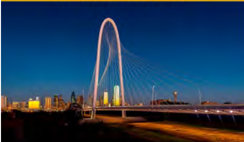
MARGARET HUNT HILL BRIDGE Santiago Calatrava/City of Dallas ■ Dallas, TX
