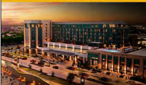
DOUG PITCOCK '49 HOTEL AND CONFERENCE CENTER NCCD-Cain Hall Redevelop I, Inc. ■ Texas A&M University, College Station, TX
