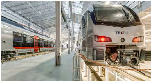
TEXRail Maintenance Facility
