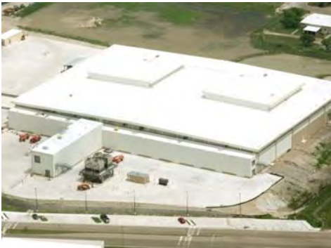
Dynamic Component Repair Facility USACE Fort Worth District
