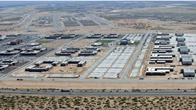
Fort Bliss Expansion Program USACE Fort Worth District
