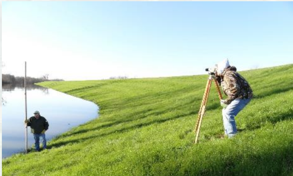
MVK: Michael Dale and Keith Gaskin of the Southeast Arkansas Lake Village Sector inspection team surveys an area of possible seepage to compare it to the river elevation.
