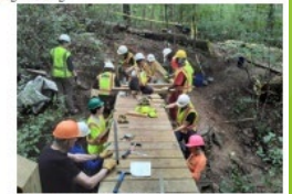
GMU EFD team during construction
