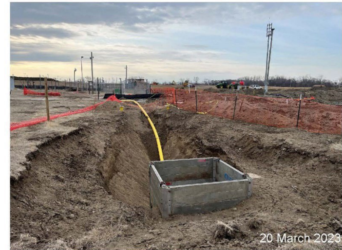
PHASE 3 – GAS LINE BORING ALONG LOOKING GLASS AVE.
