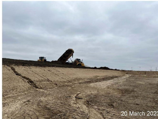
PHASE 2 – BACKFILL ON NC3 BUILDING PAD
