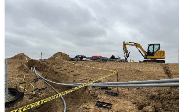
PHASE 3 – GAS LINE BORING ALONG LOOKING GLASS AVE.
