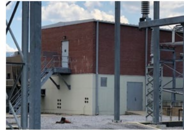
Type 2: Concrete With Steel Rebar
