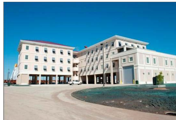
STA Sabine:: Surveyed Hurricane Harvey CAT IV
