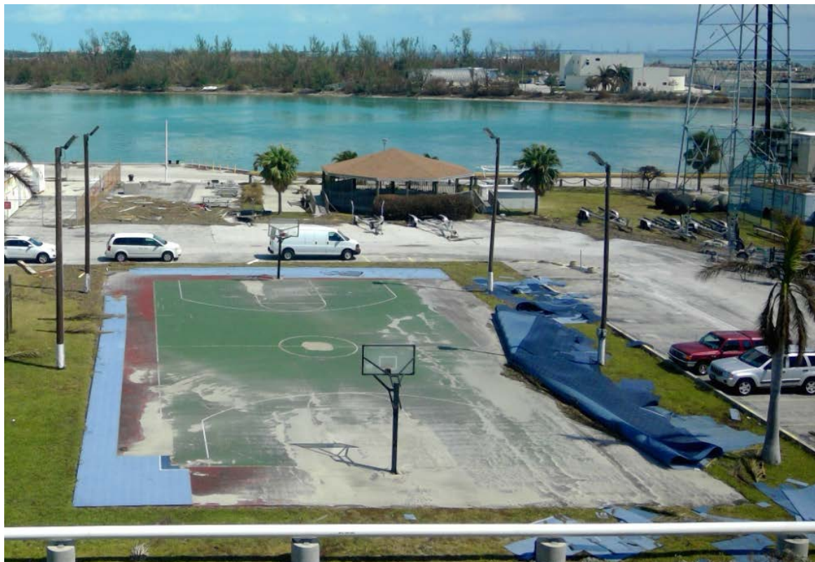
Key West – High water level and wind damage
