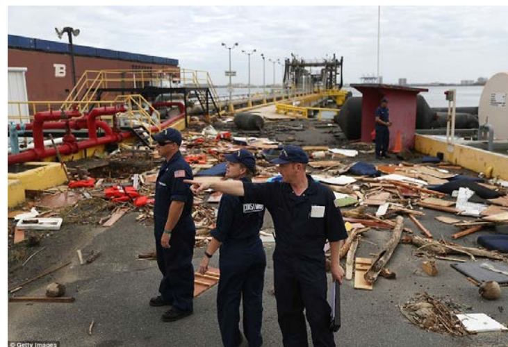
Coast Guard personnel survey the damage to an oil dock after Hurricane Maria passed through the area in San Juan
