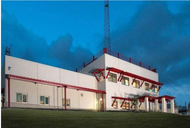
STAT Houston ...Fared well; minor roof damage
