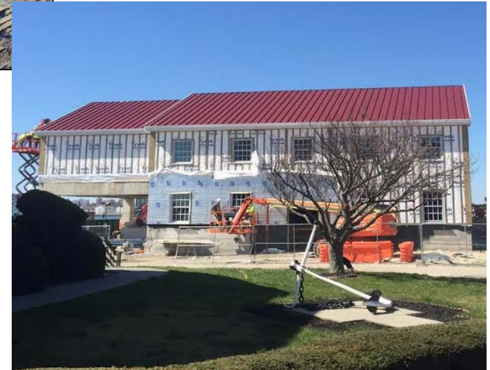
New Standing Seam Roof Atlantic City, NJ
