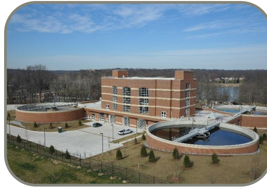
Residuals Management Project
