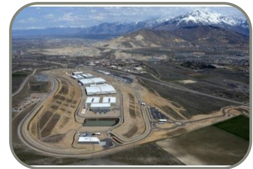
Utah Data Center
