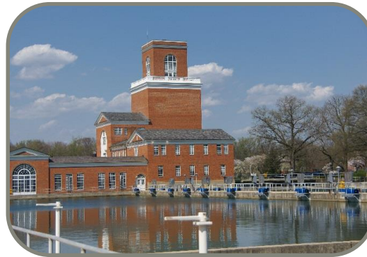
Dalecarlia Water Treatment Plant
