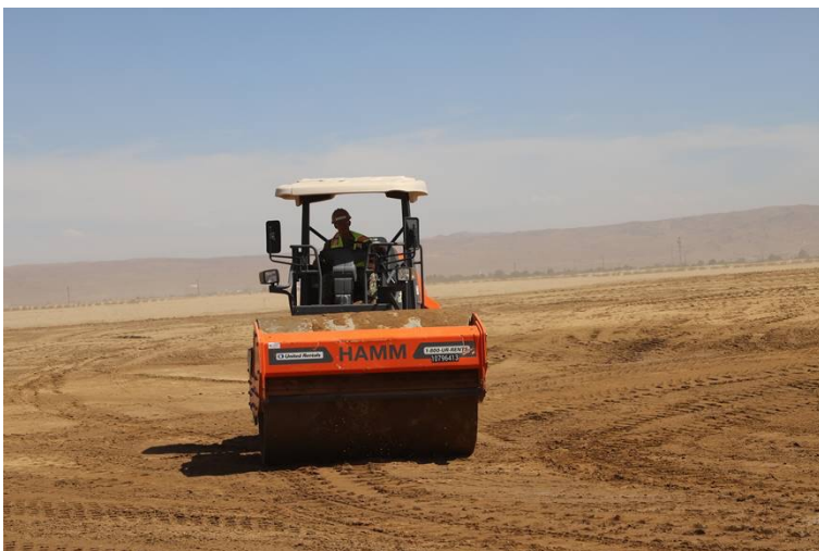
Seabee operating finish roller
