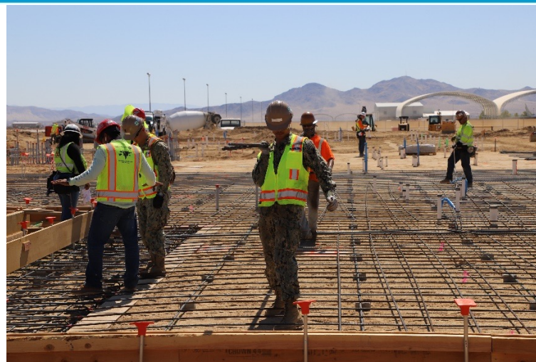
Seabees learning and supporting reinforcing bar placement for a mat foundation
