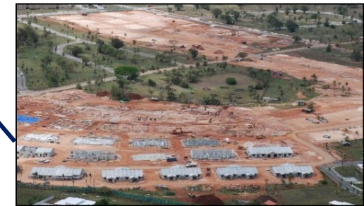
Family Housing at Andersen AFB
