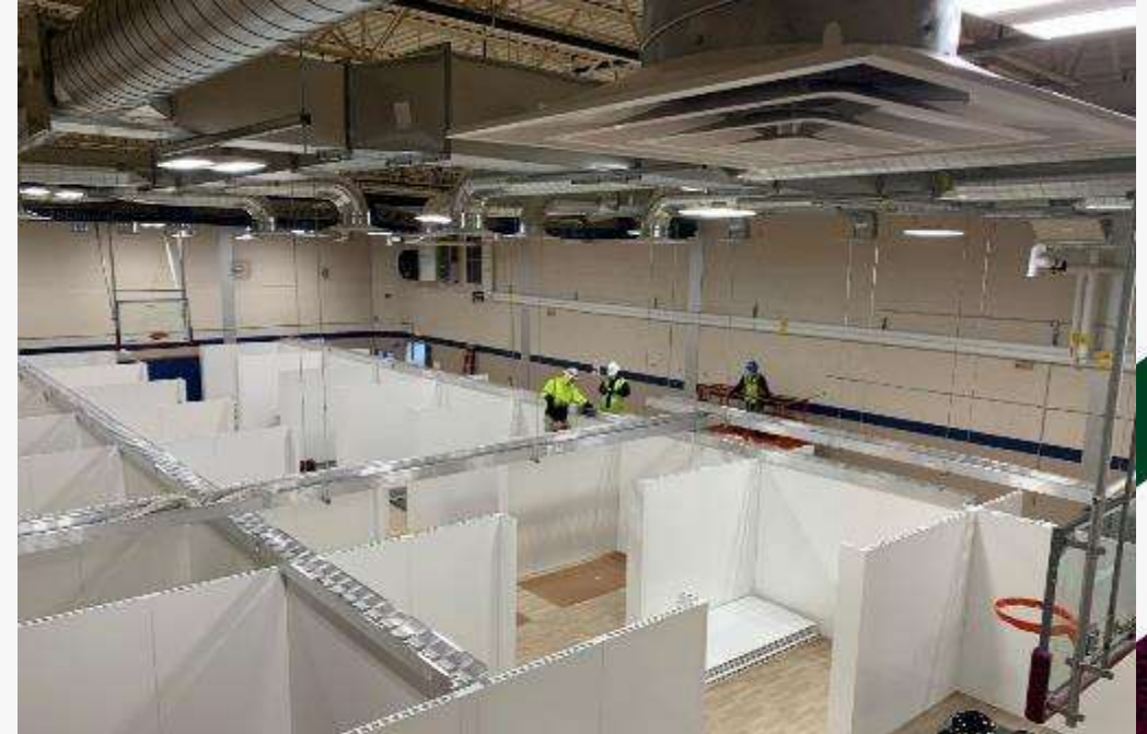
COVID-19 Alternate Care Facility Owner: USACE Philadelphia Location: New Bergen, NJ
