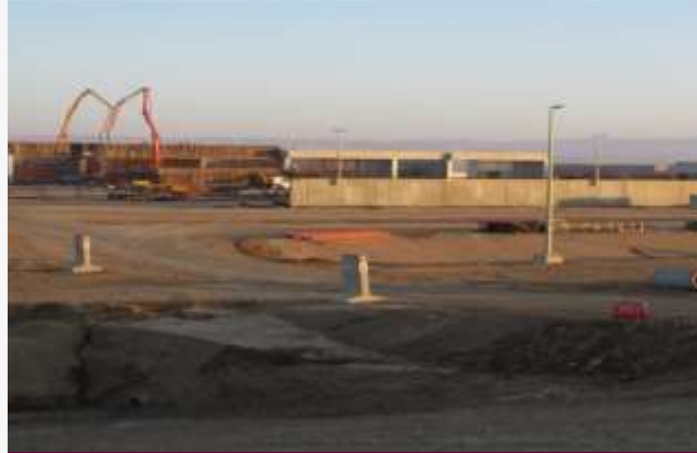
Site 417 Hardened Aircraft Shelter Owner: USACE Europe Location: Israel Value: $84,430,404
