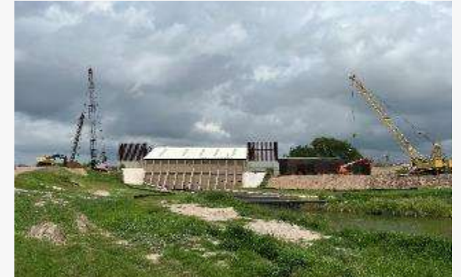
D/B Edinburg Levee Repair Owner: USIBWC Location: Edinburg, Texas Value: $6,498,887
