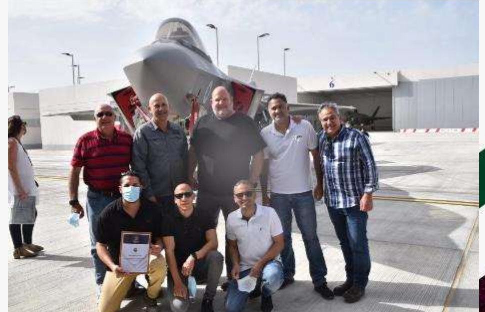
F-35 Hardened Aircraft Shelter
