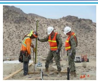
NMCB 3 with Reyes Construction measuring for batter boards onboard NAWS China Lake
