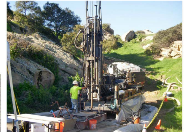
Drilling groundwater monitoring well
