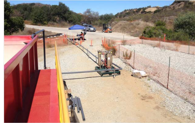
Groundwater cleanup operations
