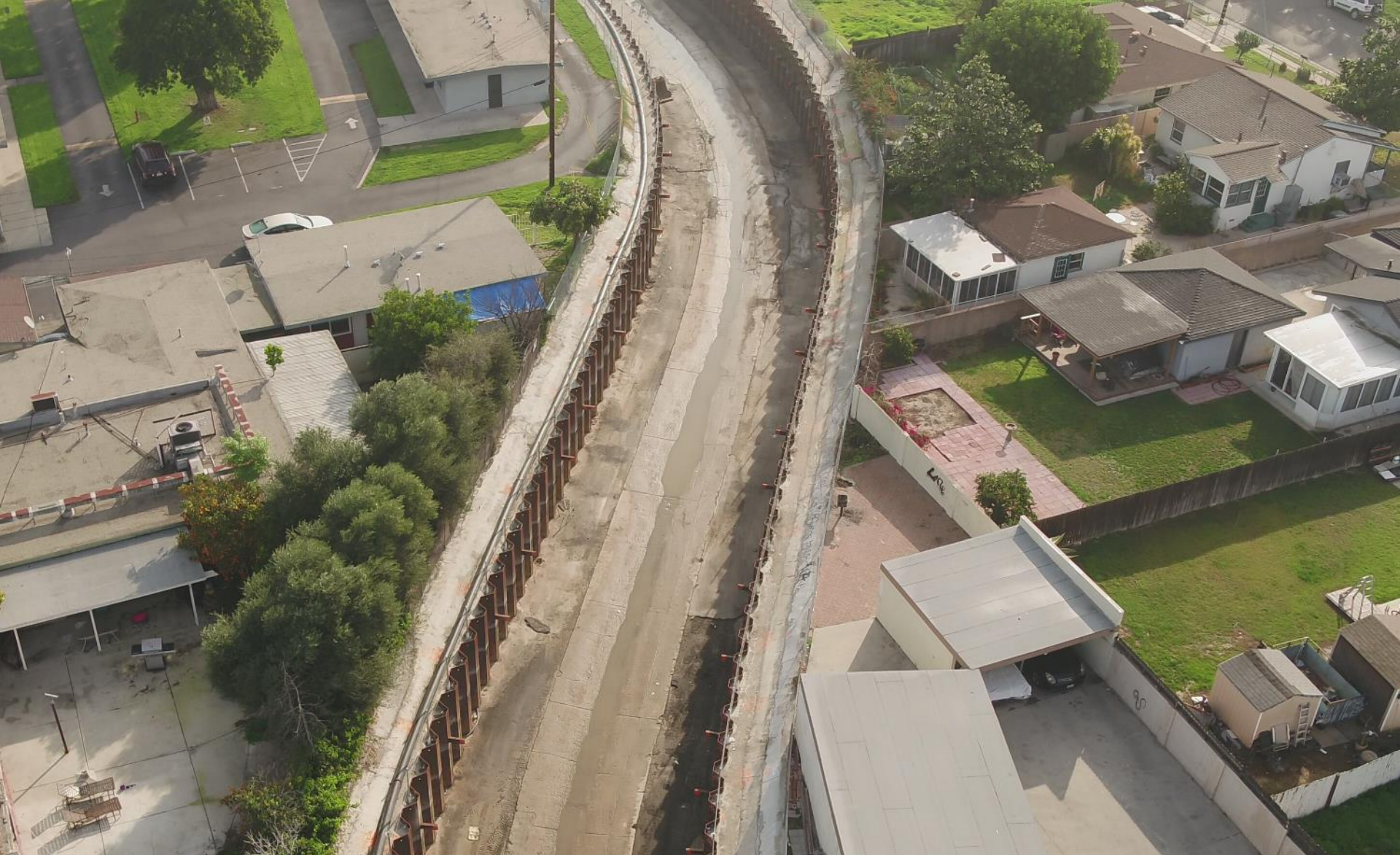
DURING CONSTRUCTION Fullerton Creek Channel- Phase 2
