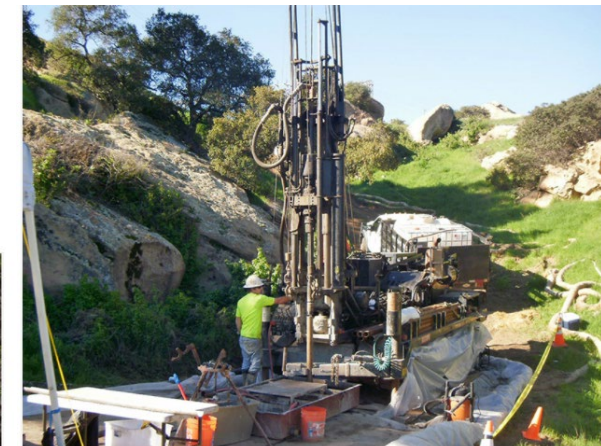
Drilling groundwater monitoring well
