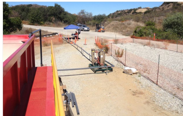
Groundwater cleanup operations
