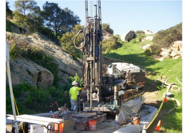
Drilling groundwater monitoring well
