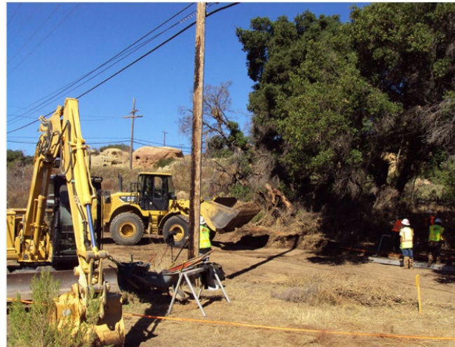
Soil cleanup operations
