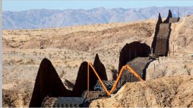
Panel Installation – El Centro – Nov 20
