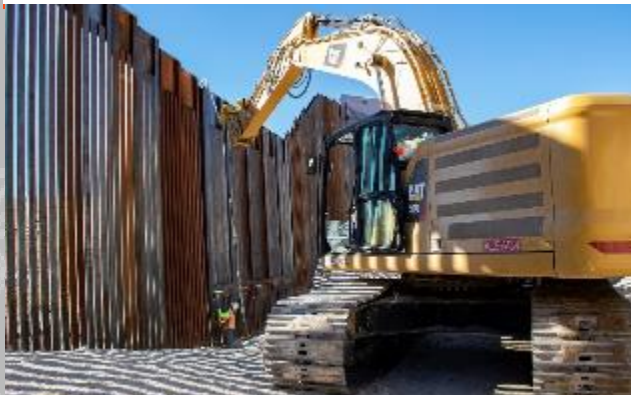
Bollard Installation – El Centro – Nov 20
