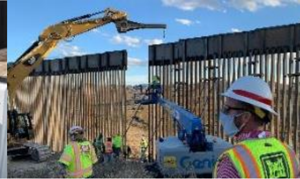
Final Panel Installation – El Paso – Dec 20
