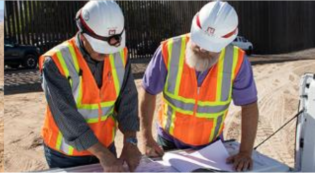
Bollard Placement – Yuma – Nov 20
