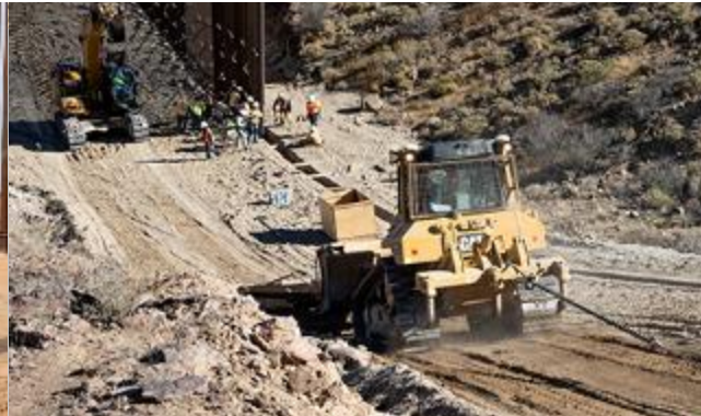
Panel Placement – San Diego – Nov 20
