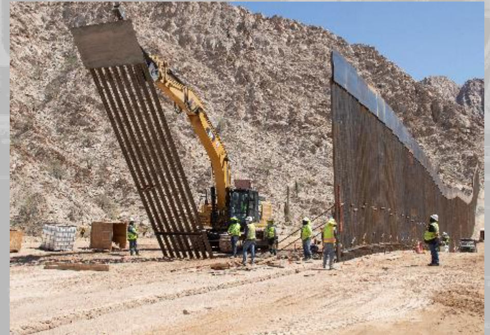
Yuma Barrier Emplacement Process in Harsh Terrain– 25 September 20
