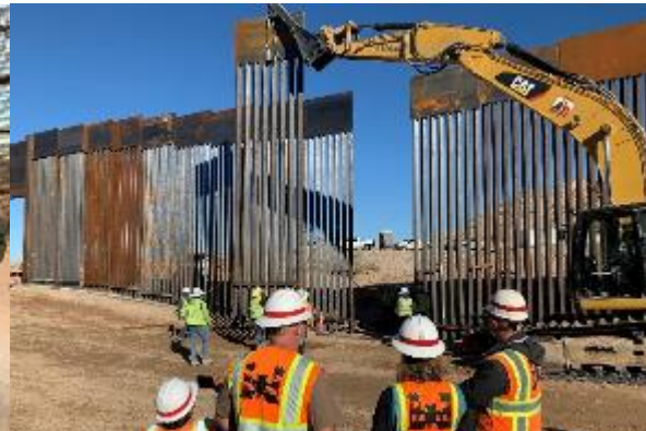
Final Panel Installation – Yuma – Dec 20
