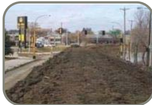
Emergency Levee Repair / Construction under PL 84-99
