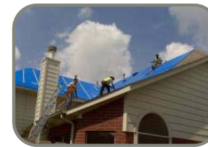
Temporary Roofing “Blue Roofs”
