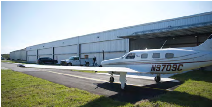
Leesburg Airport Maintenance Building Geotechnical
